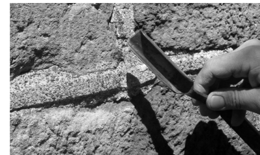
This tool is used to sculpt the distinctive ribbon pointing.
